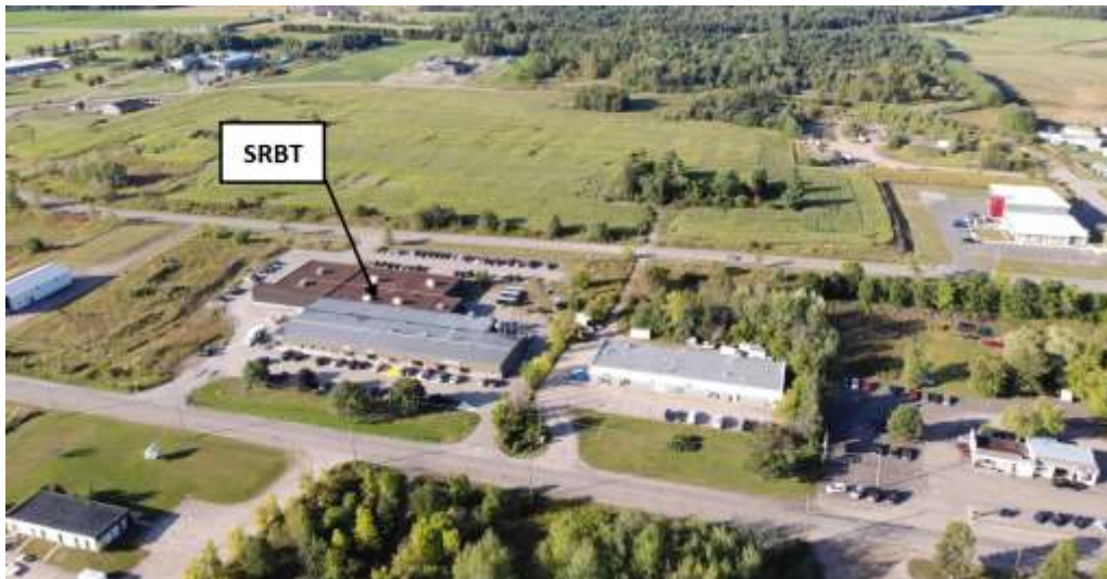
Figure 3-1: Aerial view of the SRBT facility (Source: SRTB)
