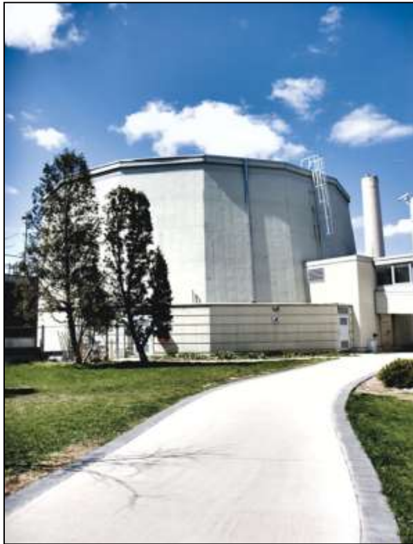
Figure 4-3: MNR containment building ( Source: MNR )
