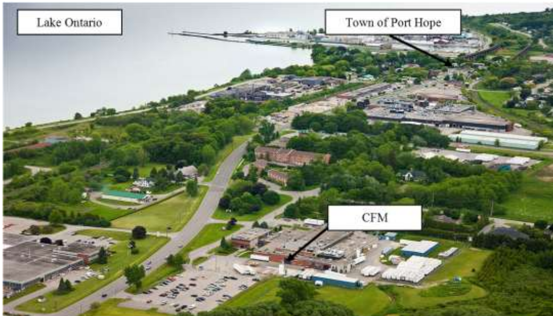
Figure 2-3: Aerial view of the CFM facility (Source: Cameco)
